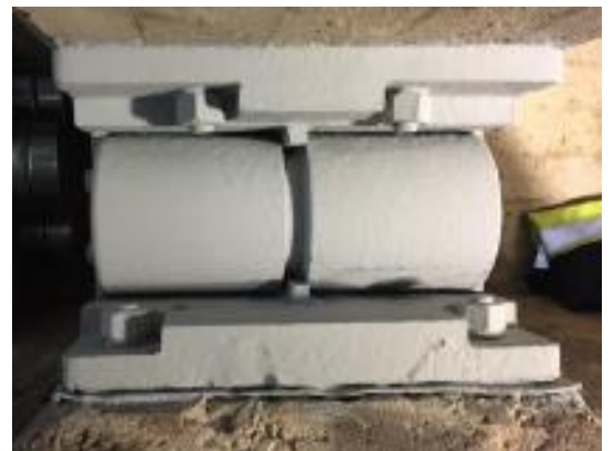
After application of ZINGA 180 µm DFT
