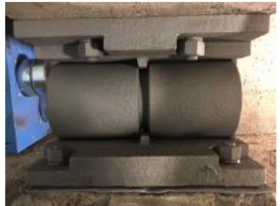
After cleaning and blasting
